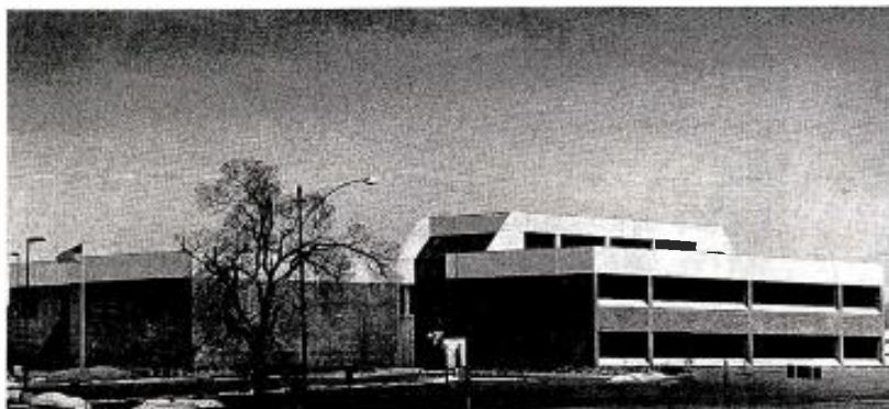
At home. Now operating out of a new $5.6 million complex is KCMO-AM-TV-KCEZ(FM) Kansas City, Mo., and Meredith Video Productions. The 56,000-square-foot building has been under construction since 1976 and is located at 4500 Johnson Drive, Fairway, Kan. Housed in the new facility are offices and studios for the three Meredith stations in addition to Meredith's production arm. The production center has two studios, computer lighting, RCA TKP-45 cameras and post production capability using 10 video-tape machines with computer editing, slow motion, animation production and remote capability.
